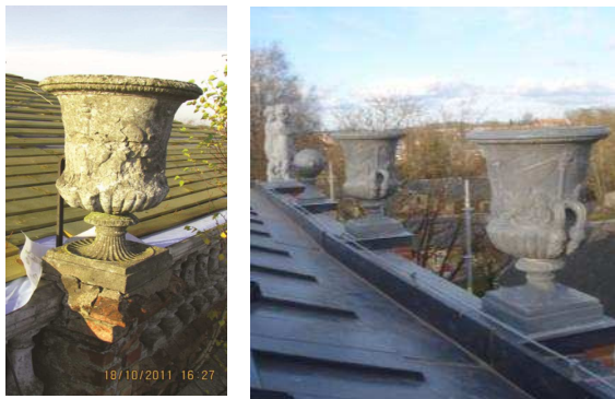
Fig. 5. Saldus Secondary School vase before reconstruction (left), reconstructed UHPCC vase (right).
