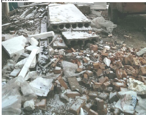
Figure 3. The view of the construction waste dump site (dump site 2)
