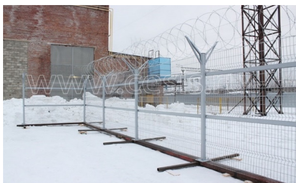
Fig. 9. An example of a reinforced similar fence, an additional stiffener, a reinforced tip (taken from the site http://www.cesis.ru )
