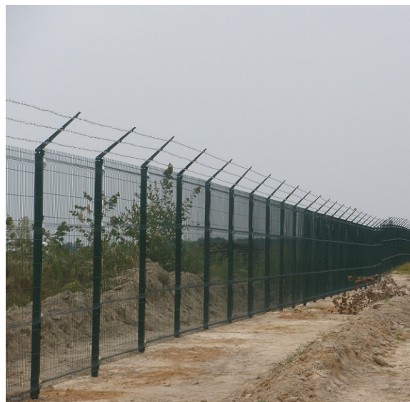
Fig. 1. View of an undamaged grating fence.
