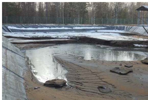
Fig. 1. Bottom sludge in a manure storage
