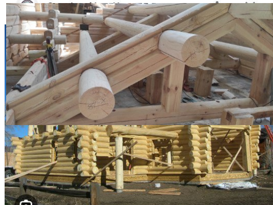
Fig. 9. The structural elements of the log house
